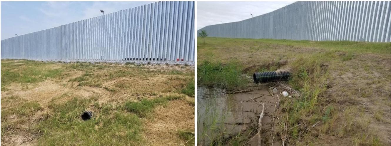
Figure 19: Drainage Culverts Installed for Fence Construction
