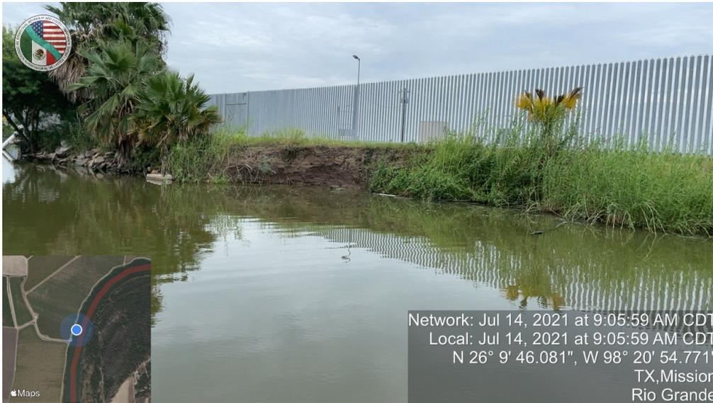
Figure 2.1. Bank erosion near fence, northeast side of fence
