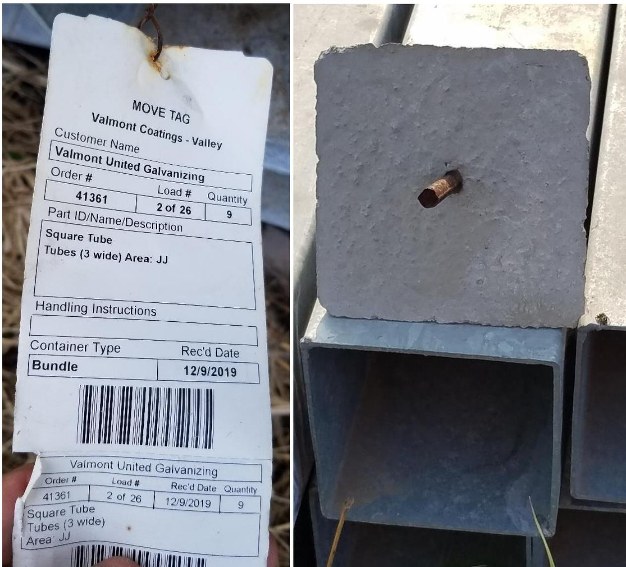
Figure 3: Shop Tag from Galvanizing, Tube Steel, and Concrete Cap with Dowel
