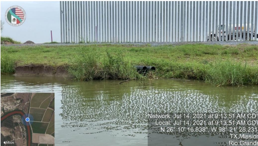
Figure 2.3. Bank caving, northwest side of fence
