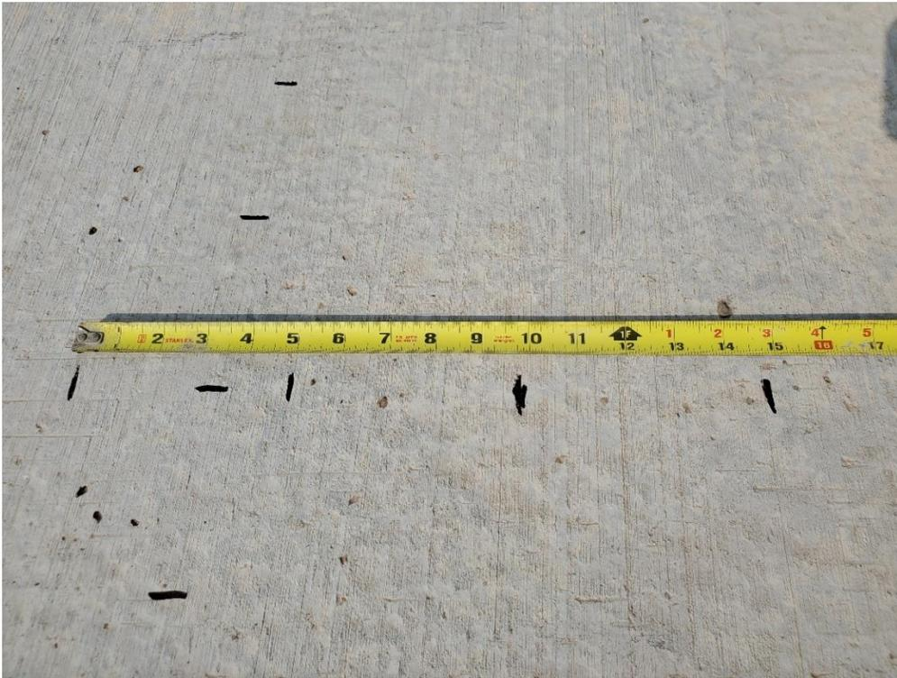
Figure 17: Rebar Spacing along footing at Approximately Every 5 Inches on Center as Determined by GPR
