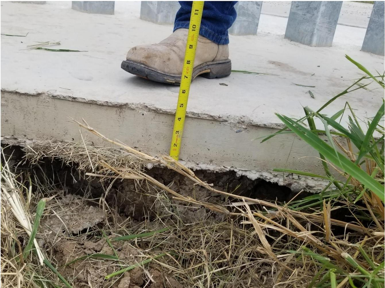
Figure 14: Footing Depth Measurement of Riverside Edge Near STA 0+00
