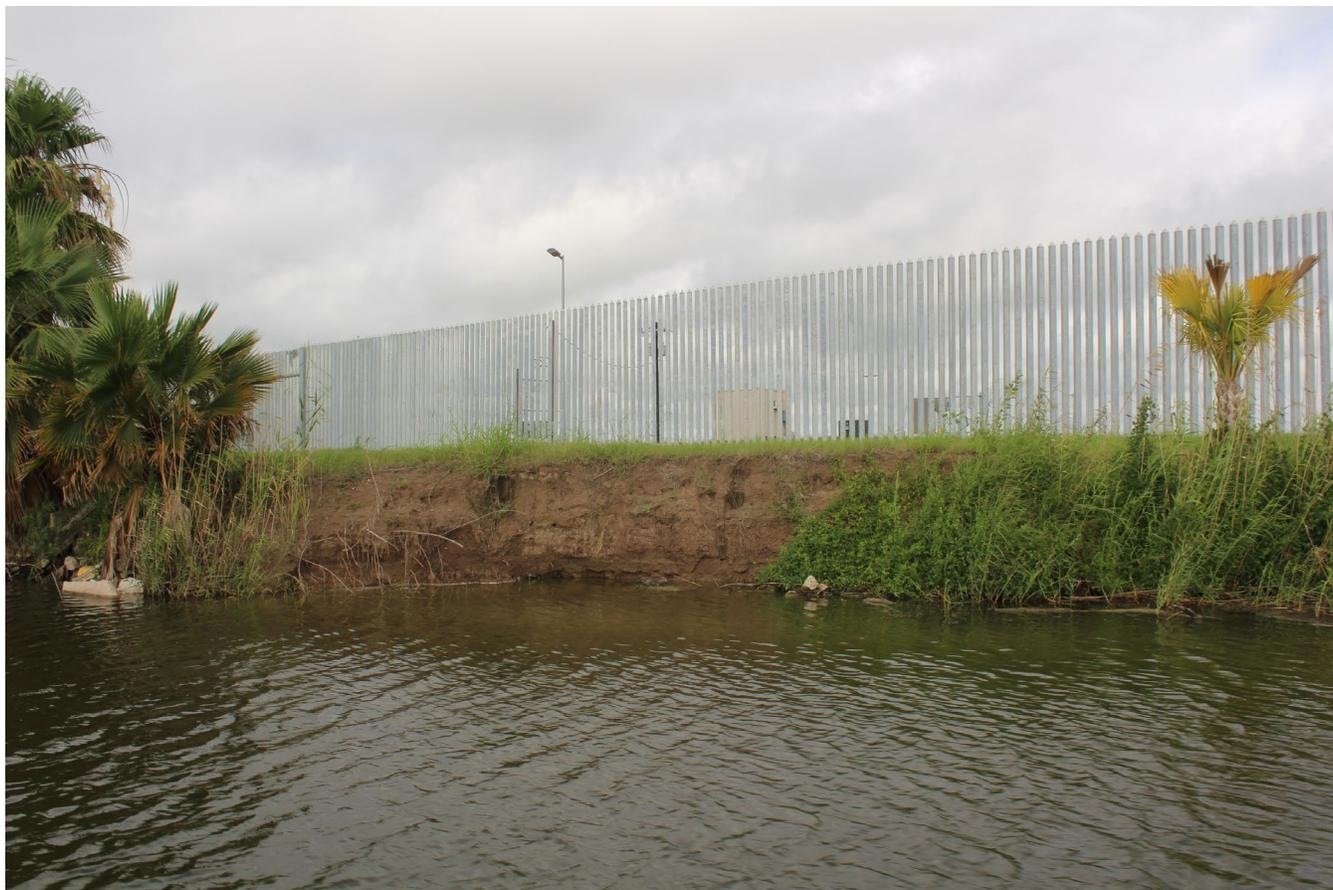
*Figure 4.35. Severe bank caving on river side of fence*
