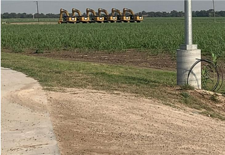
Figure 6.8. Precast shaft founded light/camera monopole
