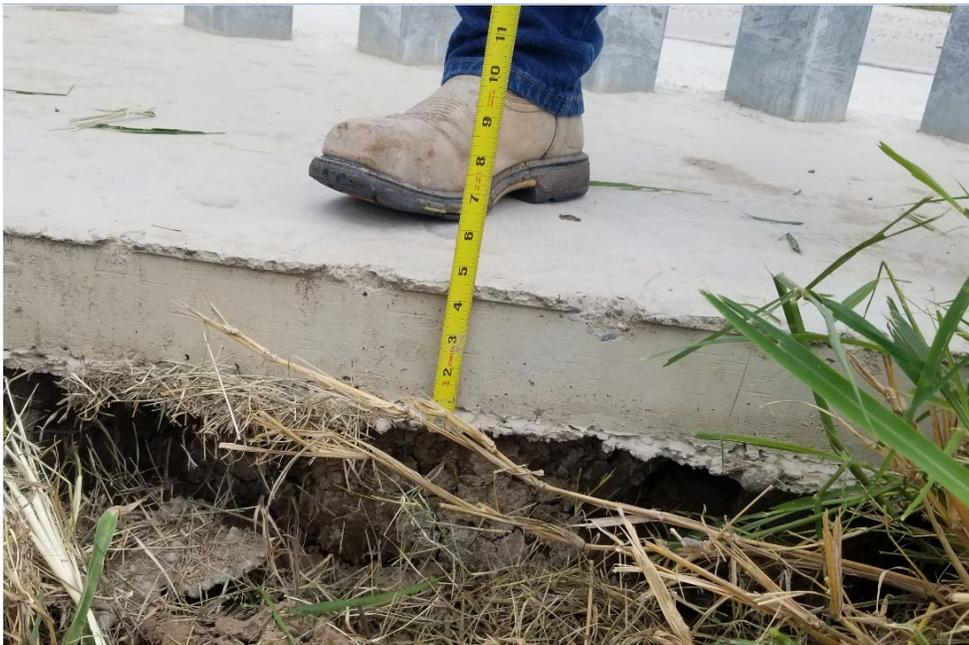
Figure 6.9. Non-conforming thickness of base foundation
