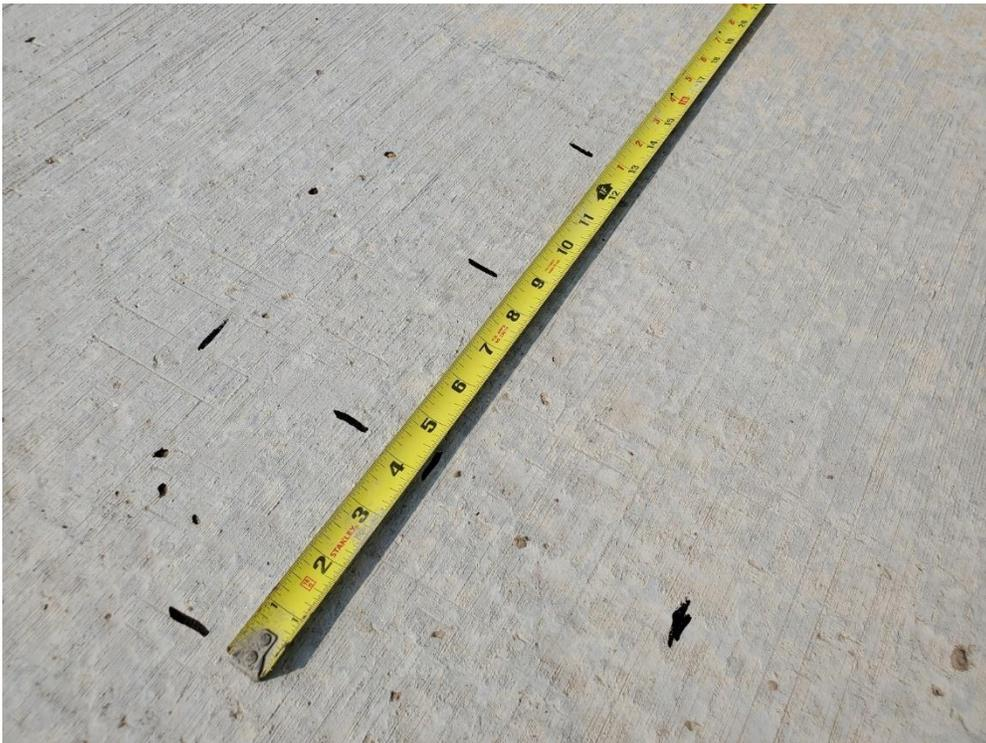
Figure 18: Rebar Spacing across footing at Approximately Every 5 Inches on Center as Determined by GPR
